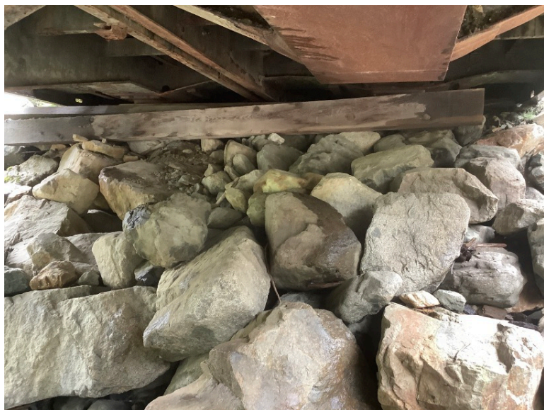
Right Bank Abutment when facing downstream
