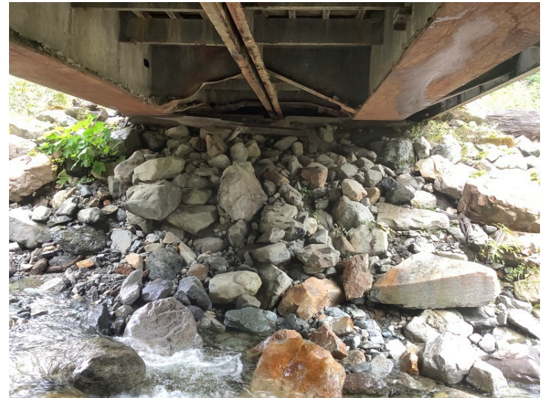
Left Bank Abutment when facing downstream
